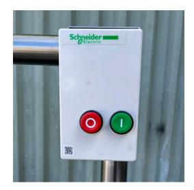
Inspect electrical terminal boxes for ingress & connections are secure (LCS, isolator & motor terminal box).
